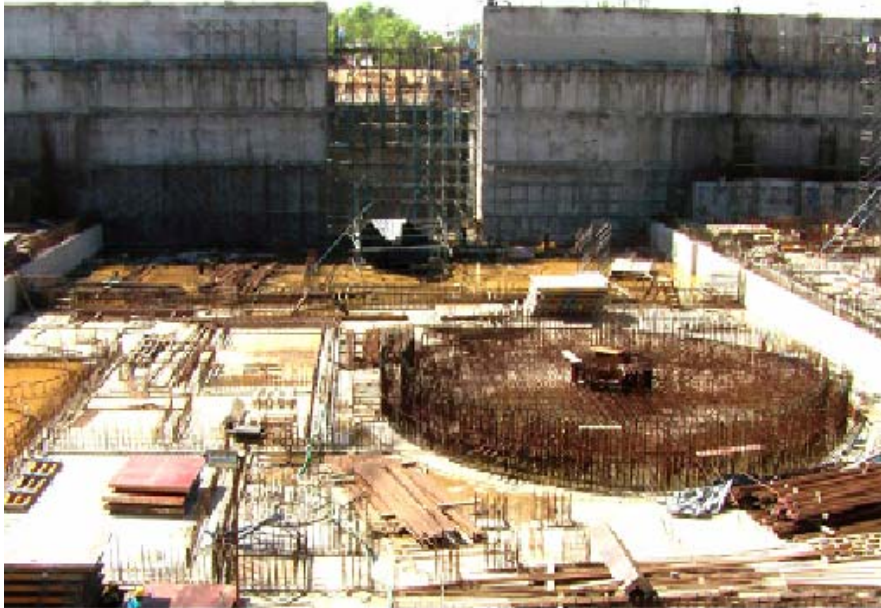
Figure 10: Construction activity at Prototype Fast Breeder Reactor, Kalpakkam, April 2006. 100
