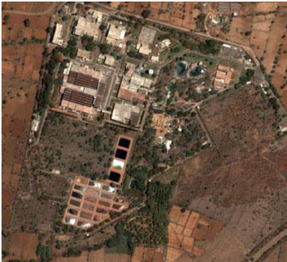
Figure 6: The centrifuge enrichment plant at Rattehalli, Mysore. 53
